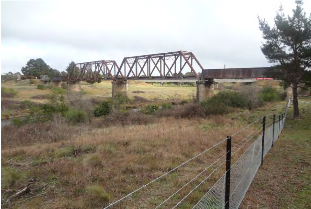
Photograph 2.5 View of the old railway bridge crossing the Wollondilly River
