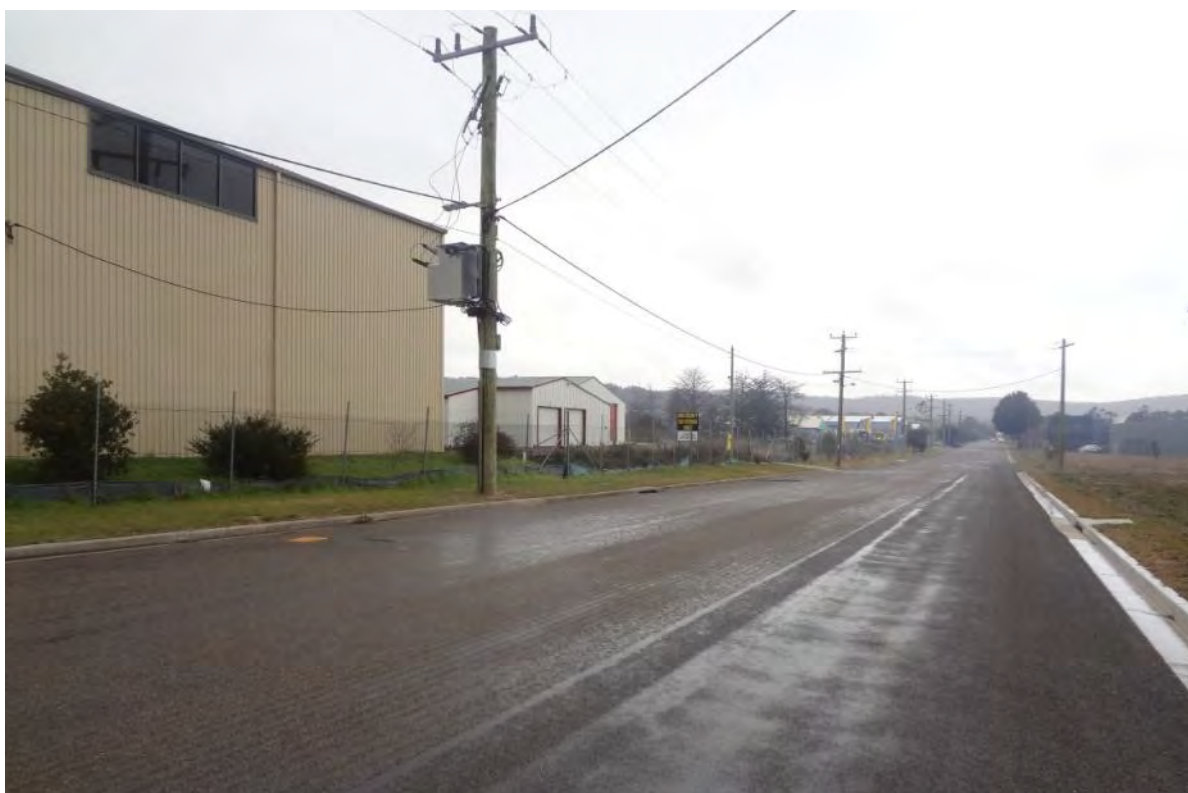
Photograph 2.4 View along Ross Street at the site frontage looking south
